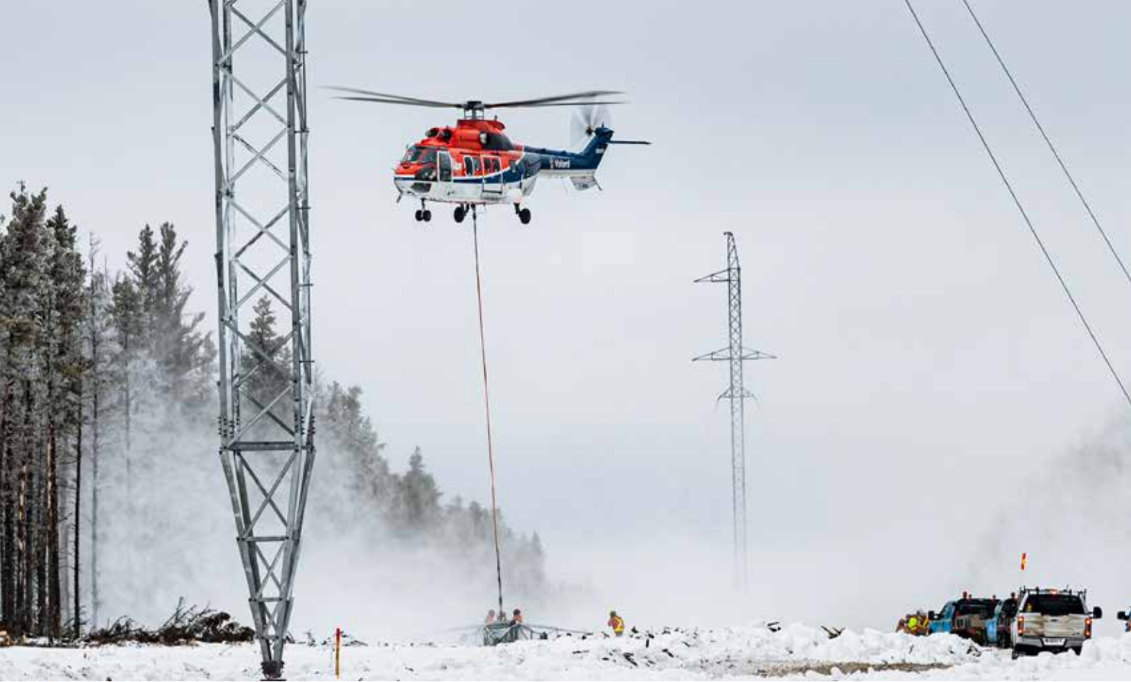
An Airbus H225 Super Puma begins to lift a steel-lattice tower from a staging area along the Watay Project right-of-way.
