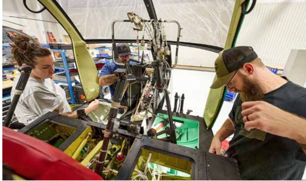
A crew installs the myriad wire harnesses, not unlike those found in any modern aircraft, as part of the in-house completions process.
